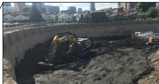
Redevelopment of former gasworks with soil stabilisation within former gas holder (images courtesy of EnGlobe)
