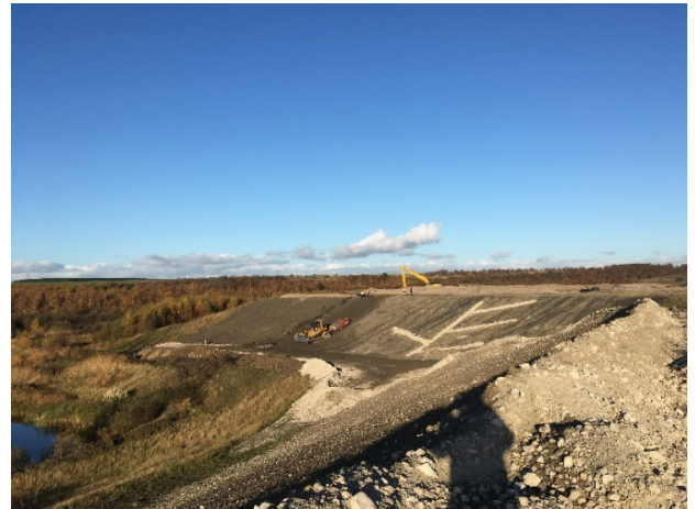
Western slope remediation showing reinstatement of lime stabilised soils (left) and new surface herringbone drain (right)
