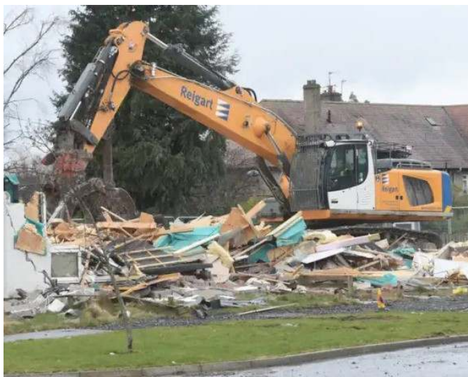
Figure 1 Demolition of Houses at Gorebridge
