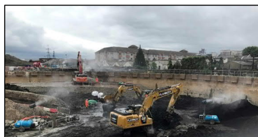
Redevelopment of former gasworks with soil stabilisation within former gas holder (images courtesy of EnGlobe)
