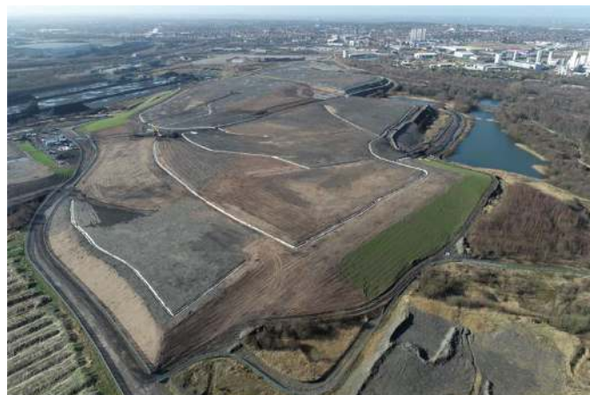
Aerial photograph of Crosby Warren Landfill in March 2022 showing completed capping works
