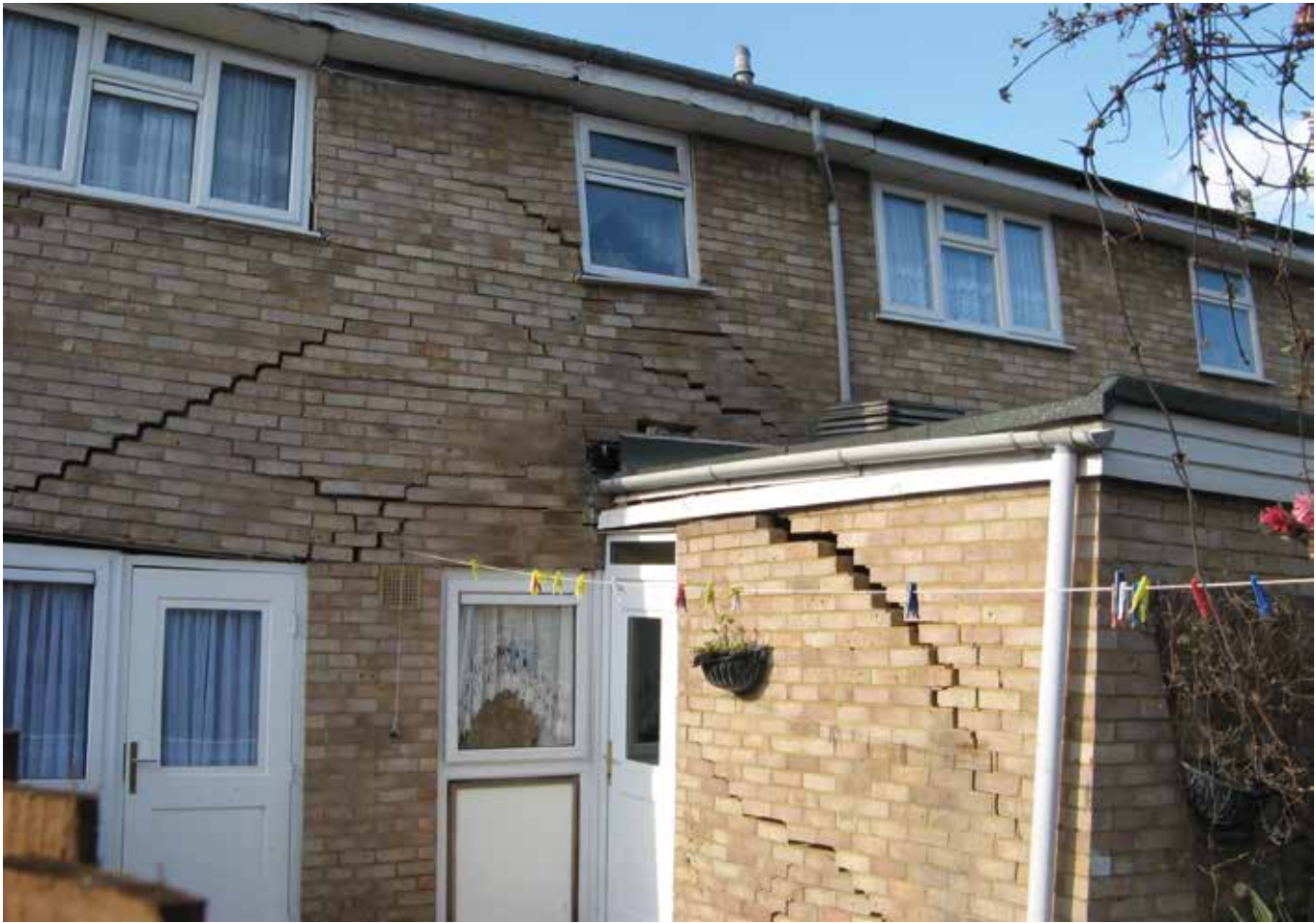
▲ Figure 2. Damage to housing caused by a sink hole. (© RSK)
