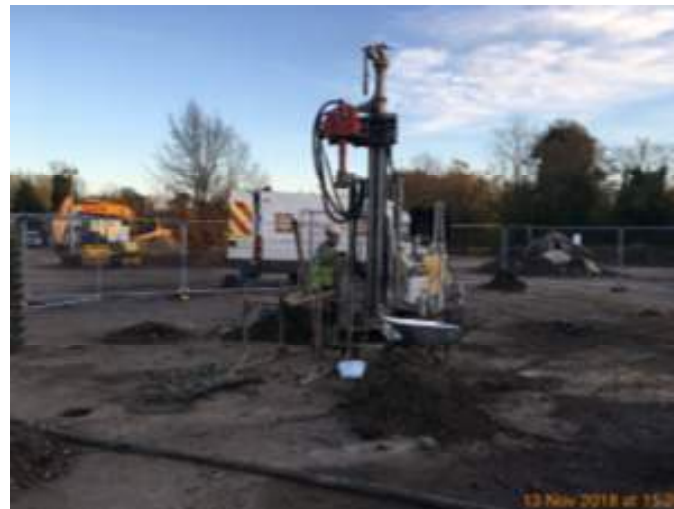
Rotary Drilling of 30nr Remediation Wells
