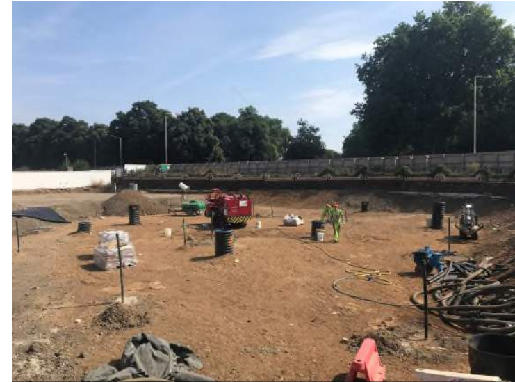
Petrocleanze Injection into LNAPL Source Zone (3-4mbgl)
