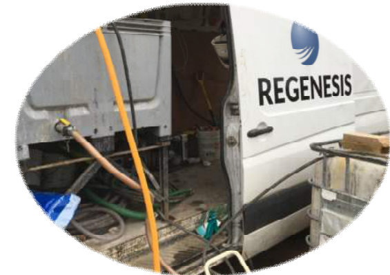
Multi-phase ISCO injection down wells
