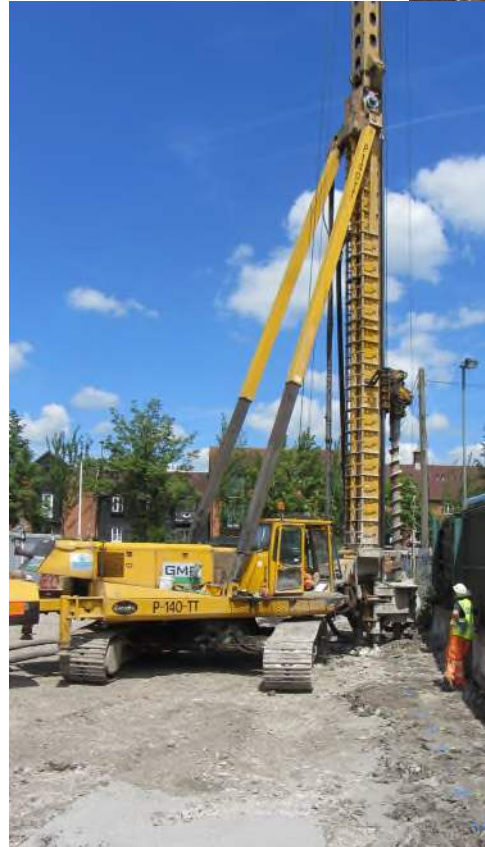
Soil Mixed Cutoff Barrier
