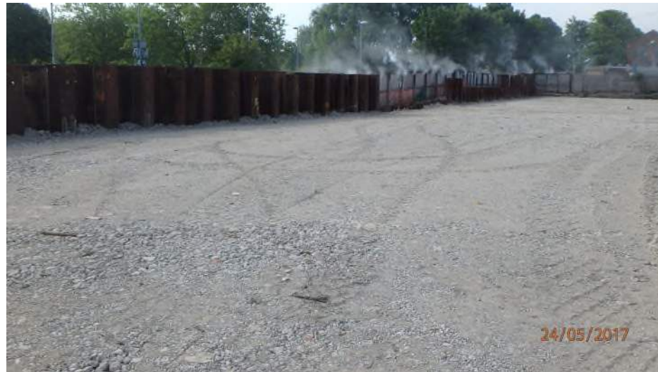
Completed Development Platform
