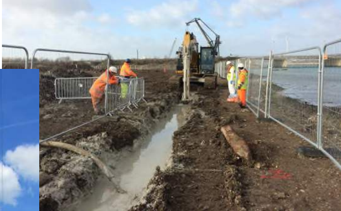
Slurry Wall Cutoff Barrier
