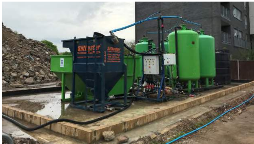
Direct-push injection of 3DMe Substrate into aquifer (4-7mbgl)
