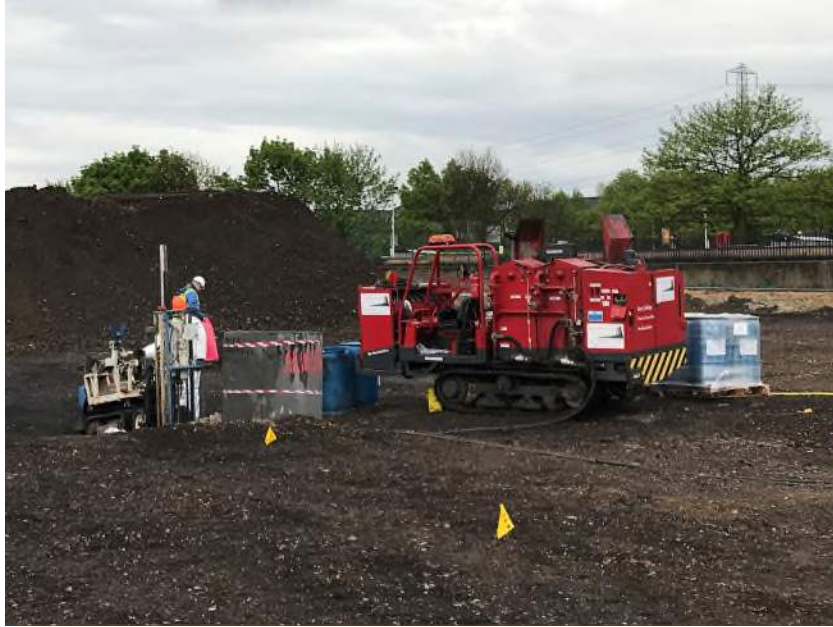
Direct-push injection of 3DMe Substrate into aquifer (4-7mbgl)
