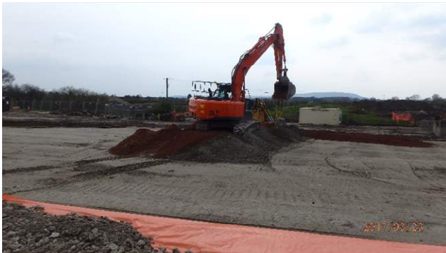
Placement of orange marker geotextile
