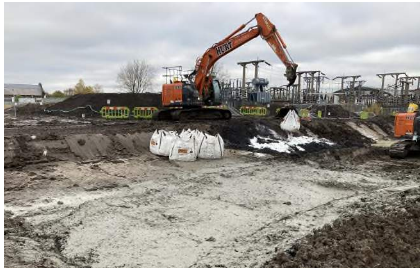
Chemox-Stabilisation/Solification (CSS)
