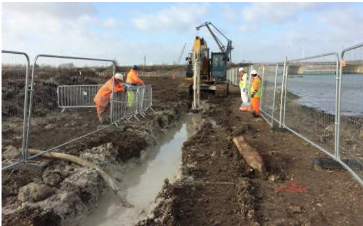
Slurry Cutoff Barrier Installation
