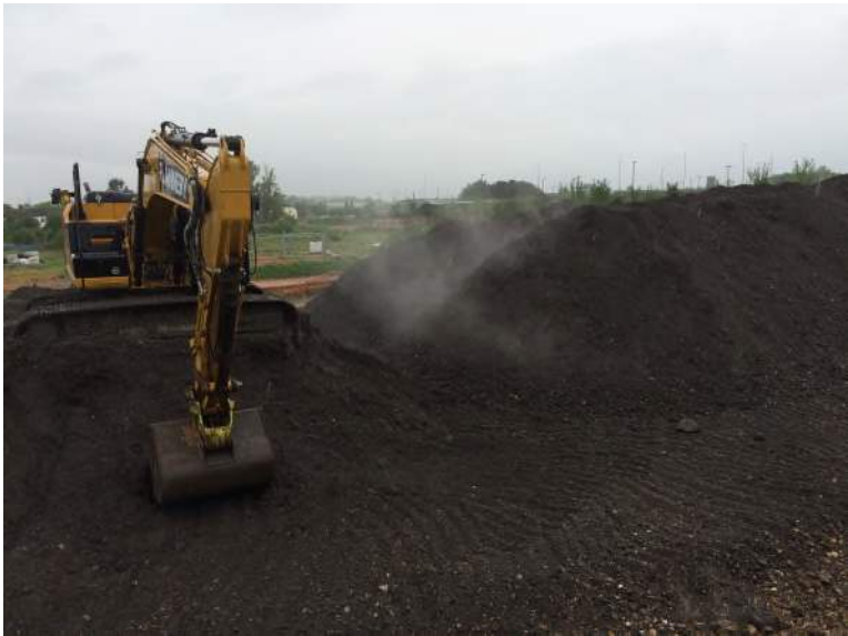
Bioremediation of Hydrocarbon Contaminated Soils
