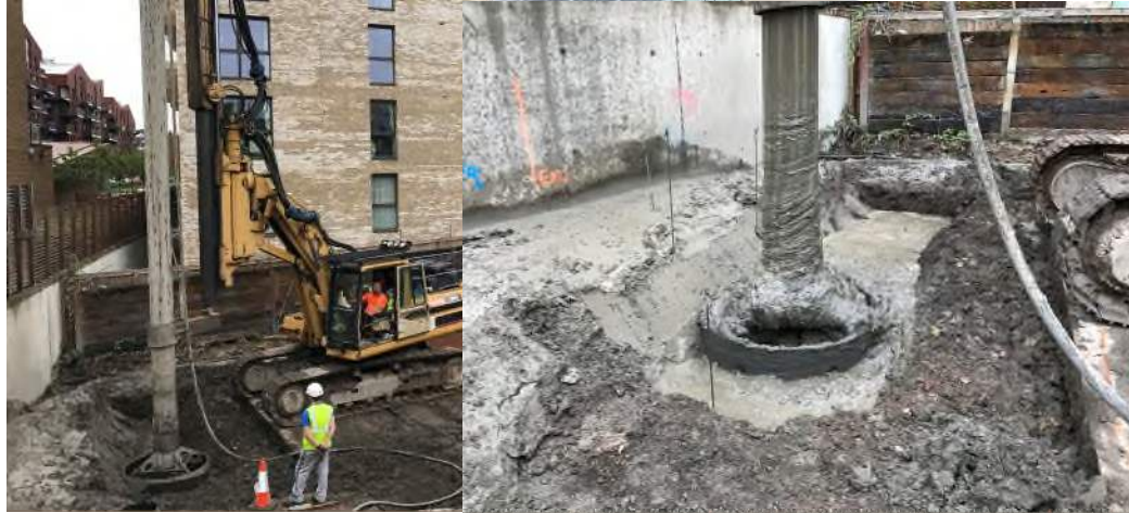
In-situ Stabilisation/Solidification
