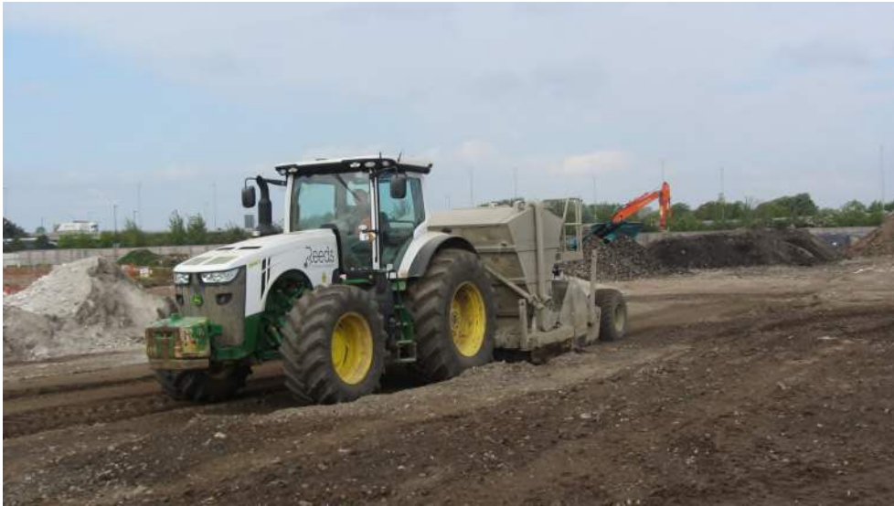
Cement stabilisation of site-won fill
