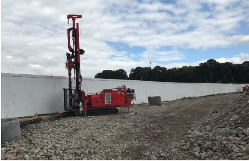
Drilling 30nr Injection Wells Along Boundary
