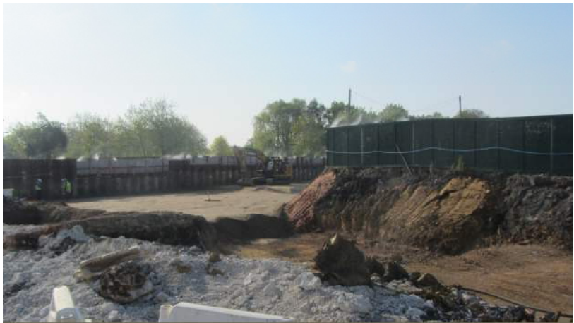
Deep excavation of Made Ground
