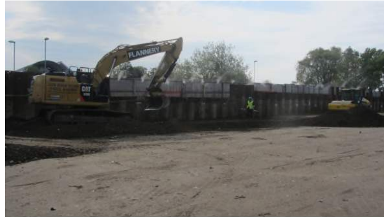
Placement/compaction of S/S Materials
