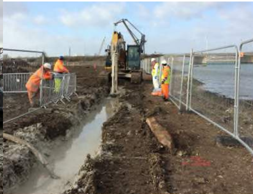
Slurry cutoff-barriers
