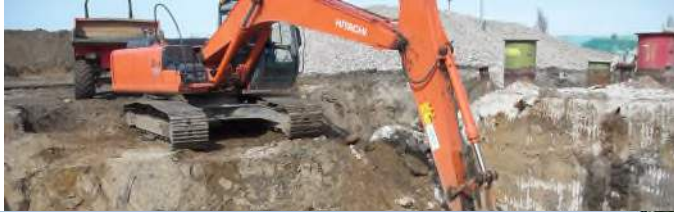
Excavation of Source
